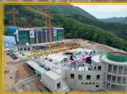
Ridge Beam Placement, April 2021
